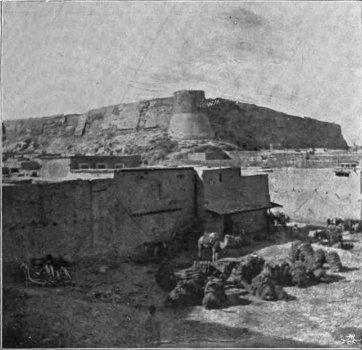
THE CITADEL IN BOKHARA, SAID TO HAVE BEEN BUILT BY ALP-ARSLAN, THE PERSIAN KING. IT IS WITHIN THIS CITADEL THAT THE PALACE OF THE AMEER IS LOCATED
