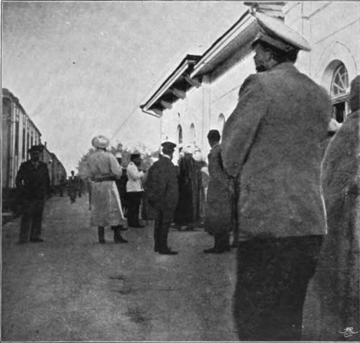
STATION AT BAIROM-ALI ON TRANS-CASPIAN RAILWAY, ON THE ROAD TO BOKHARA
