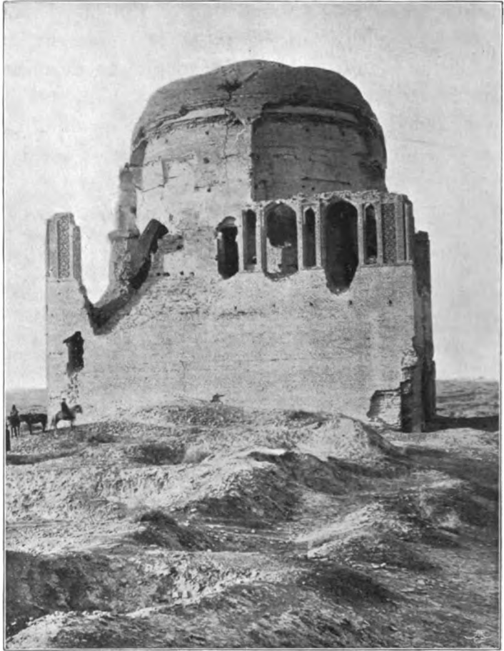
RUINED MOSQUE OF THE SULTAN SANJARE
